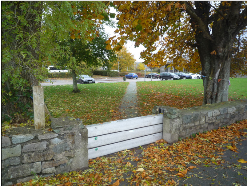
P1 – Gap in existing wave wall to be filled and tarmac footpath lifted within RPA Of tree numbers 96 & 97
