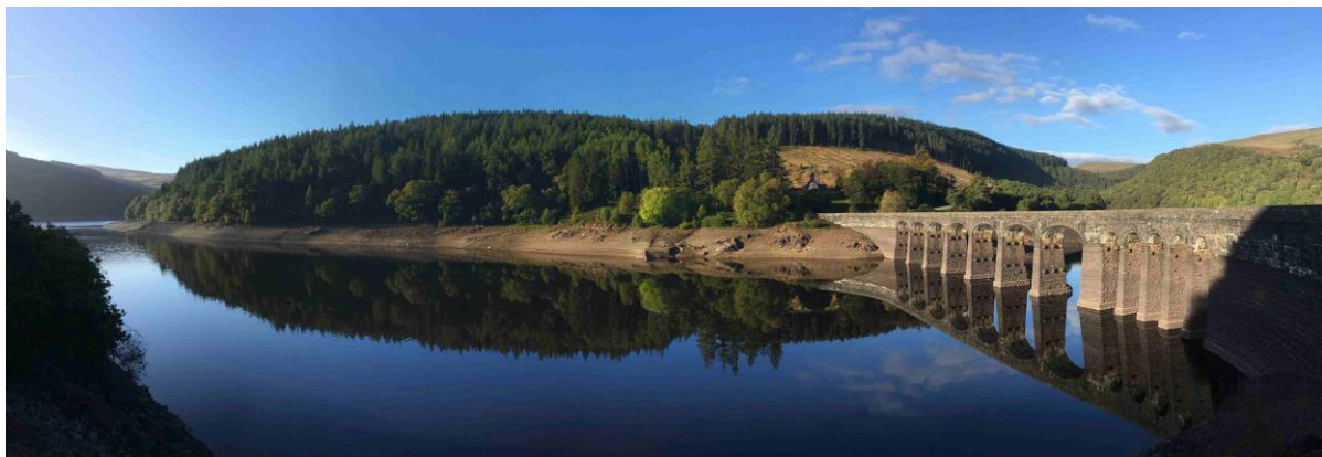
Figure 88 Caban Coch Reservoir site photo; from the north-west shore at Garreg Ddu dam, looking south-east.
