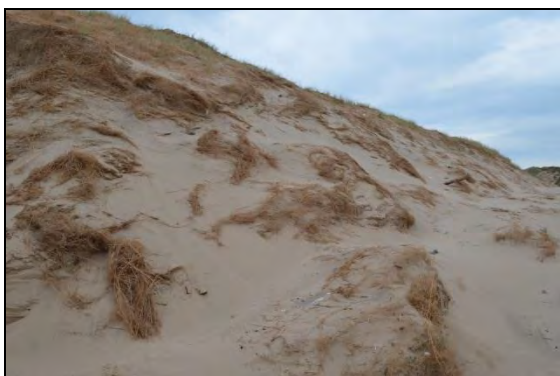
22) Detail of slope angle at notch number 9.
