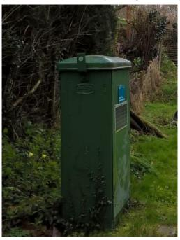
An example of a bespoke solar telemetry kiosk, which will provide a higher voltage output and reduce the need for site visits by NRW operations staff.
