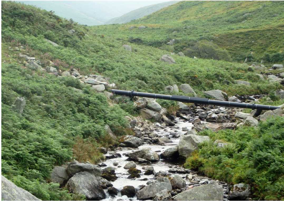
The penstock crossing the stream, 2017.
