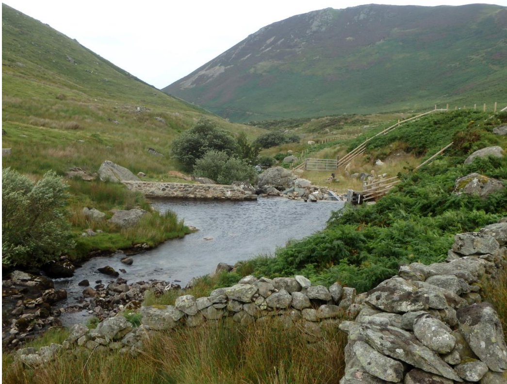
Looking downstream from constructed intake in 2017.
