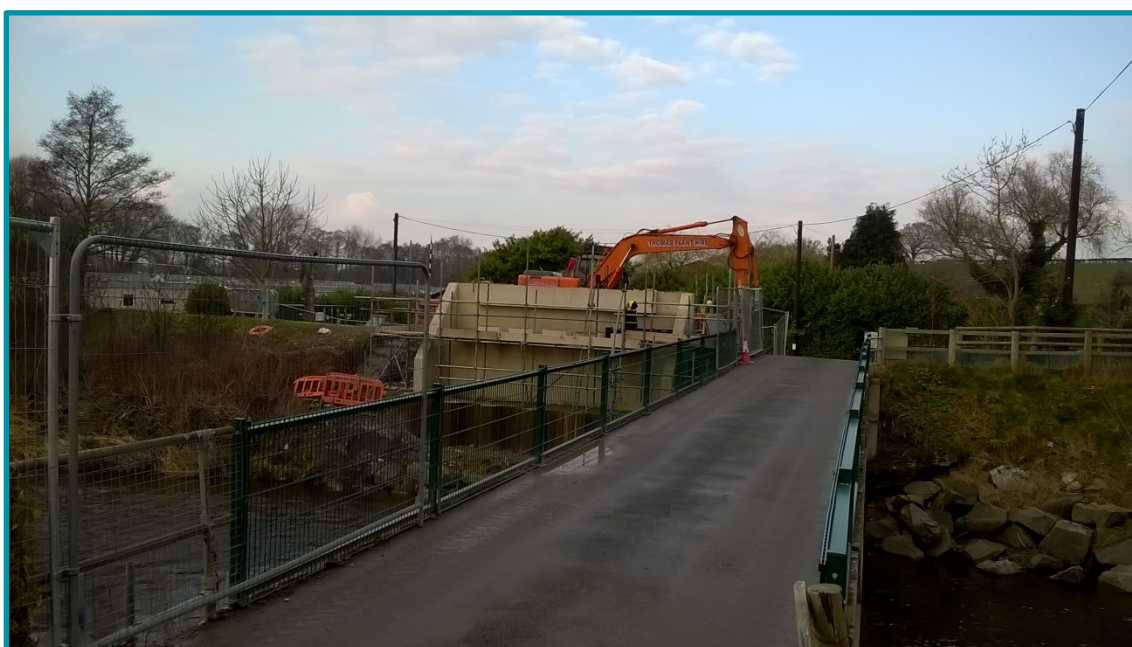
Figure 2 – work in progress to replace Spring Gardens Bridge
